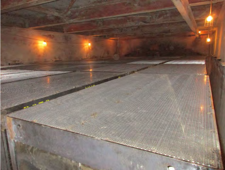
Wygen 3 U5 SCR with air cannons and secondary LPA screens
