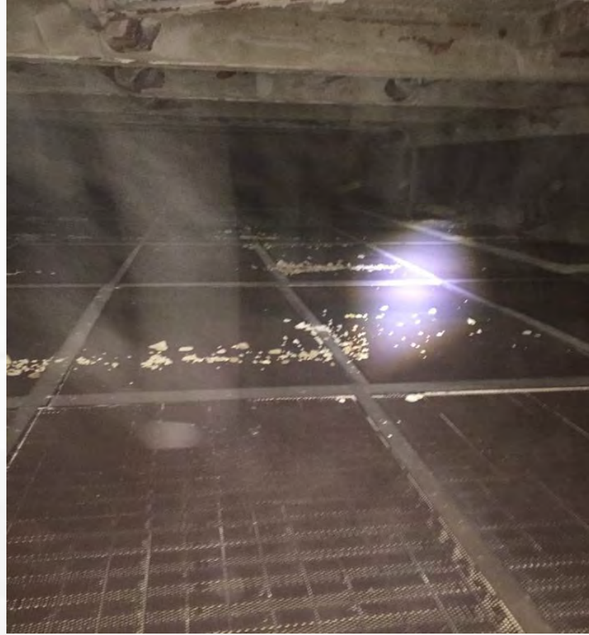
Wygen 3 U5 SCR reactor after secondary screens, LPA screen modifications and air cannons
