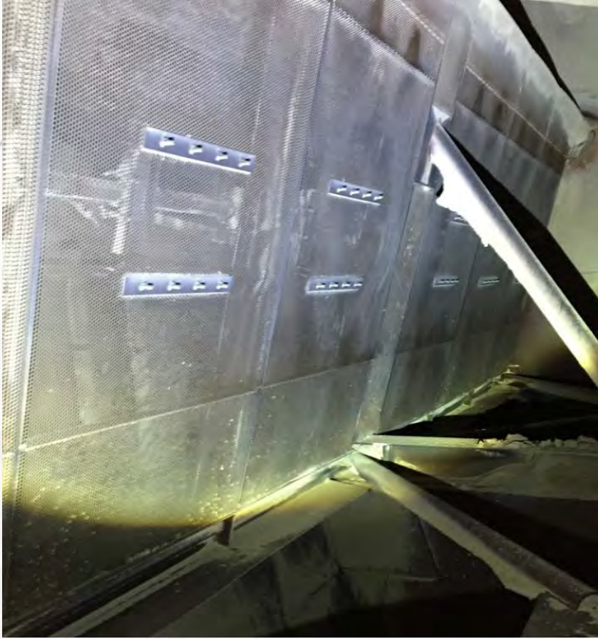
Wygen 3 U5 LPA screen after LPA screen air cannon installation
