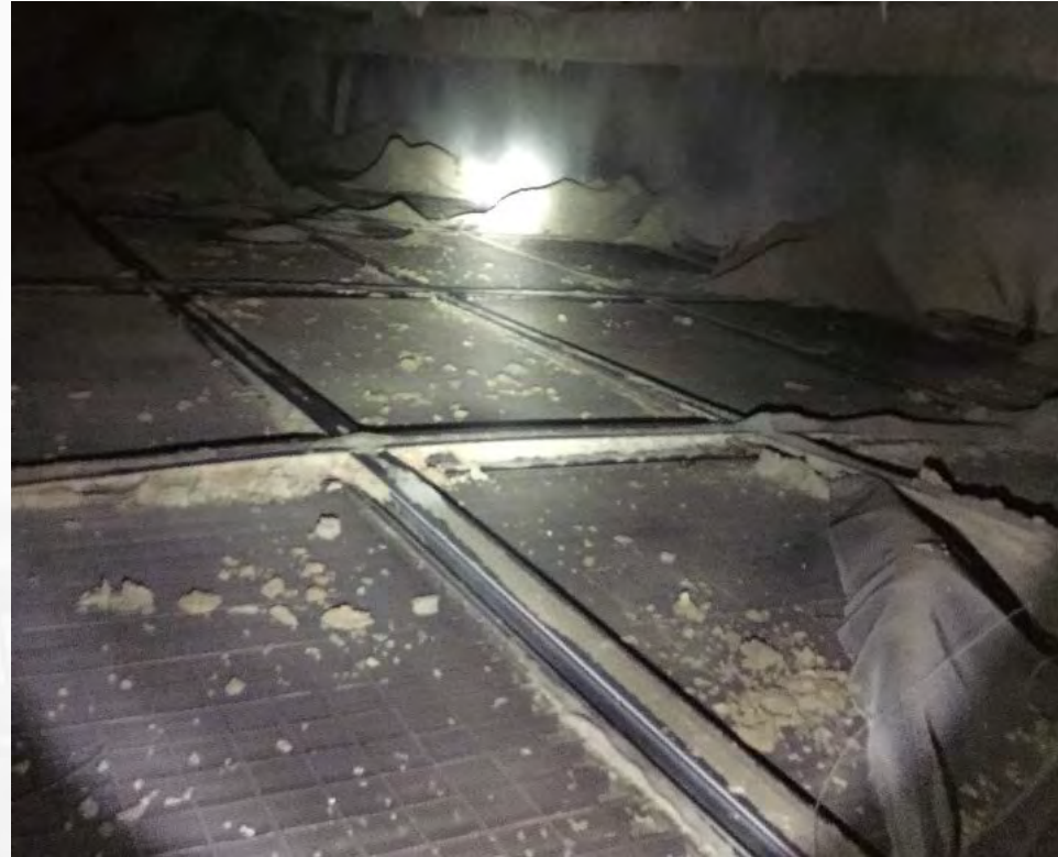
Wygen 3 U5 Bottom Layer with Wire Mesh Catalyst Screens
