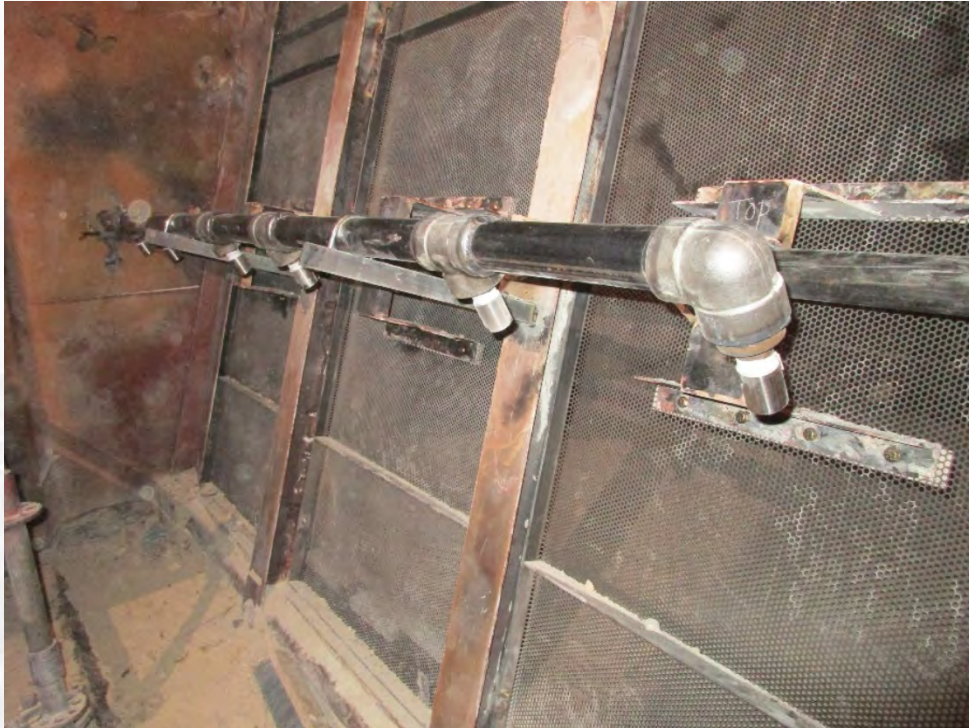
Wygen 3 U5 LPA screen air cannon cleaning system during installation
