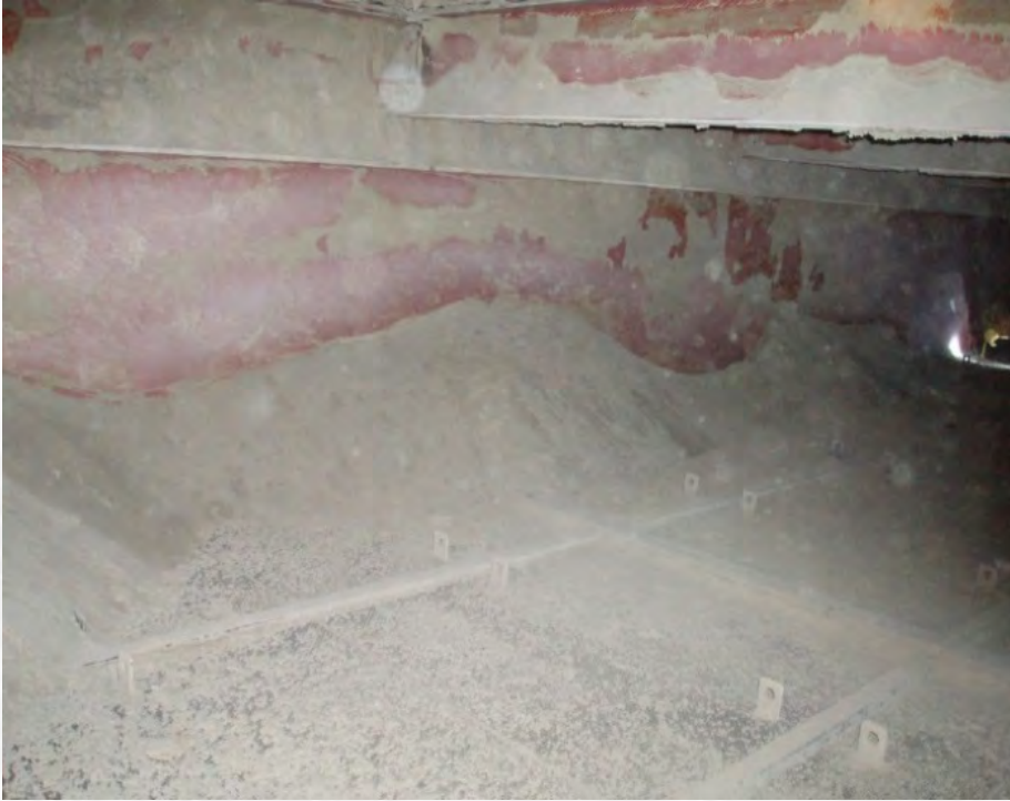
Wygen 3 U5 SCR reactor before secondary screens, LPA screen modifications and air cannons
