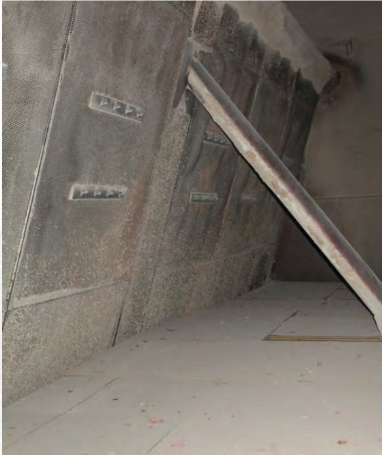
Wygen 3 U5 LPA screen prior to air cannon installation
